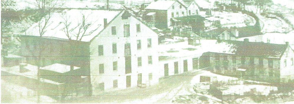
Mills along Indian Creek near 65th Street and Havenford Avenue - 1915. Photograph by John W. Eddfield. Note the rows of houses built up to the edge of the valley. This mill, situated at the confluence of the east and west branches of Indian Creek, was eventually torn down, and the playing fields in Morris Park were built on the filled and leveled location. Free Library of Philadelphia Print & Picture Collection
