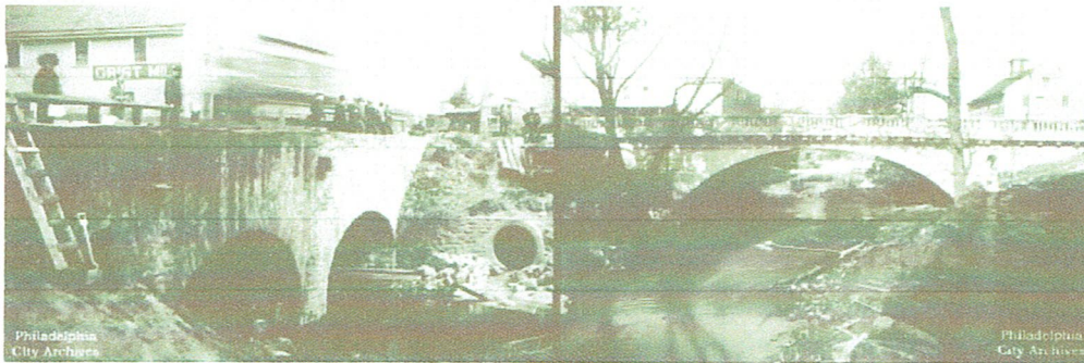
Woodland Avenue at Cobbs Creek, looking upstream. Old bridge, left, on October 22, 1908. Note the open sewer emptying its contents into the creek. This old bridge was replaced by a new concrete bridge (left), shown in 1909. Philadelphia City Archives
